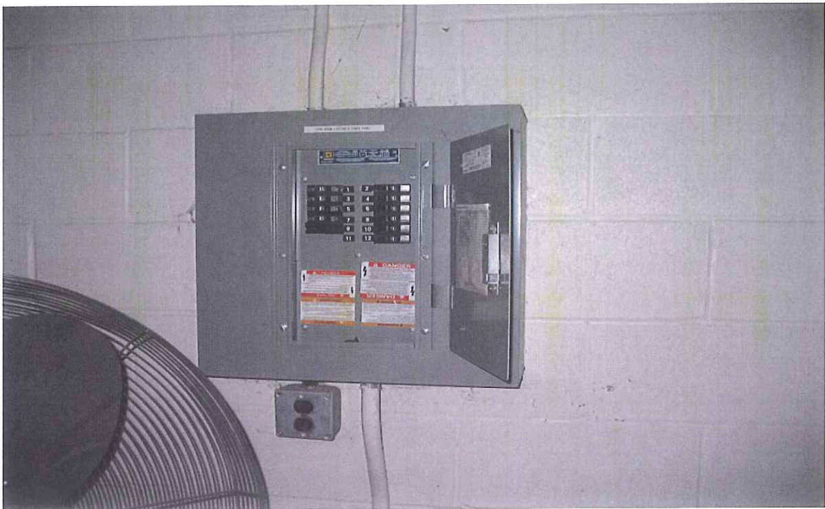
PUMP ROOM LIGHTING & POWER PANEL
